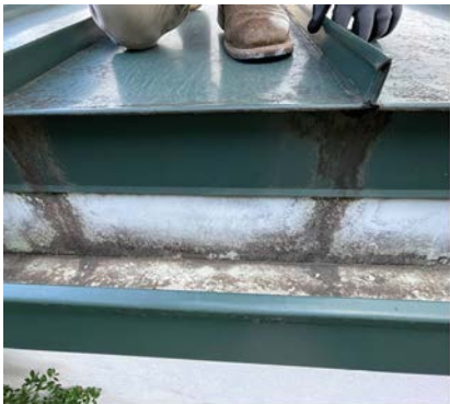
An example of a well-installed standing-seam double-lock system.
