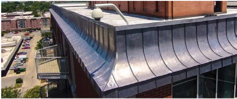
A concave, lead-coated, double-lock system on a student housing center
